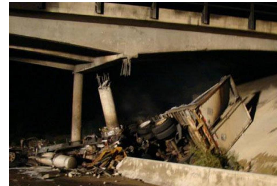
Fig.1. Failure modes of bridge column
