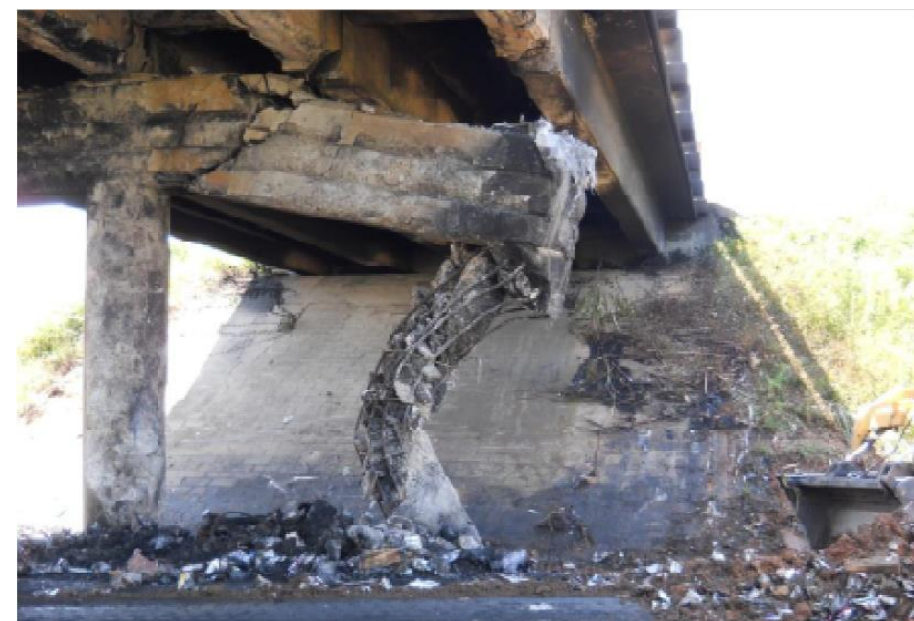
Fig.1. Failure modes of bridge column
